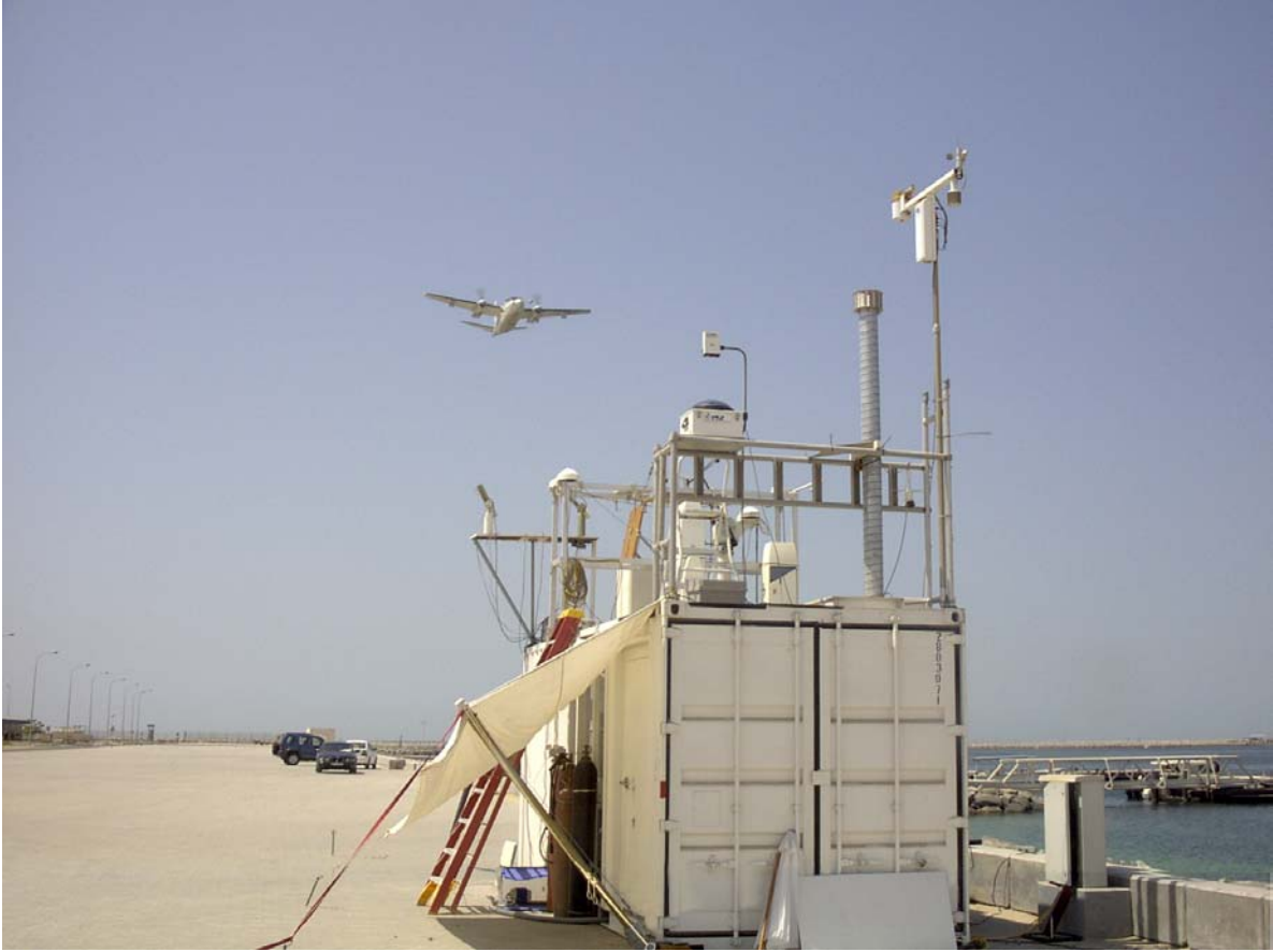
Figure I.1. Overview of MAARCO container with outboard radiation and meteorology equipment with Aerocommander over-flight
