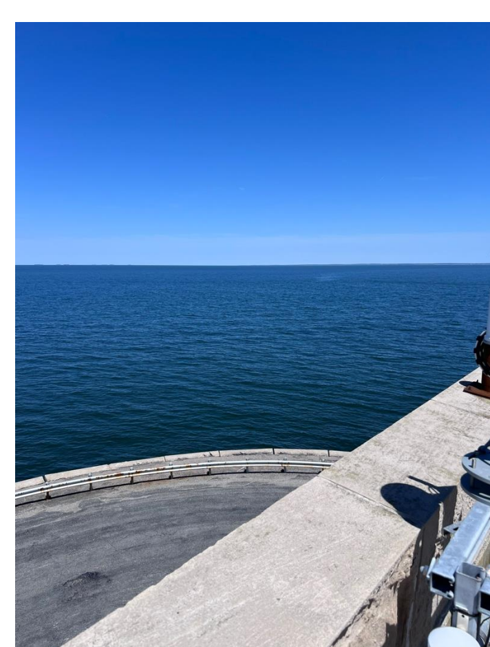
Instrument view towards the North.
